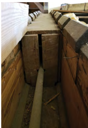
Fig. 2 Image of one of the steel beams supporting the Grand Reading Room provided by BBI Construction Management, Inc. during the 2020-21 restoration of the south facing exterior of Smathers Library.
