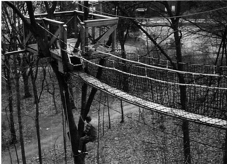
FIGURE 1. Photograph of walkway during construction at The EcoTarium, Worcester, MA.
