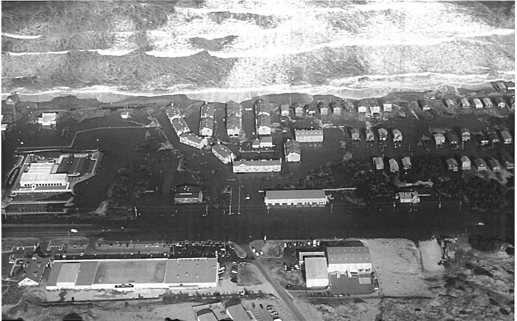
Kitty Hawk, North Carolina. View looking east on 31 October, 1991 during the "Halloween" storm. Waves are washing across the "beach" road Hwy 12. The flood waters also cut off the "by-pass" road Hwy 158 which is the only other north-south route on the island. The ocean-front building in the upper left is the U.S. Life Saving Station #6 built before the turn of the century. The building was moved about a mile southwest shortly after the storm. (Photograph by Carl Miller, WES/CERC Field Research Facility, Duck, North Carolina).
