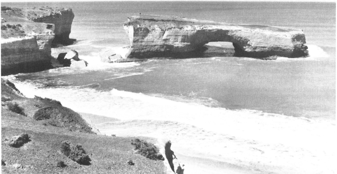
London Bridge (a double arch structure near Port Campbell, Victoria, Australia) as it was in March 1977 (upper photo). The inner arch collapsed into the sea at 7:45pm on 15 January 1990 (lower photo), just after two people had walked across it to the outer arch. They were rescued by police helicopter three hours later. Although small pieces of rock had fallen from the inner arch from time to time, the collapse was sudden and unexpected. (Courtesy of Eric C.F. Bird).
