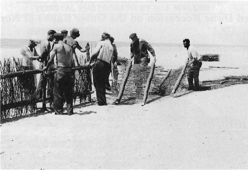
Figure 1. Installation of sand fencing along the Outer Banks of North Carolina in the 1930s.
