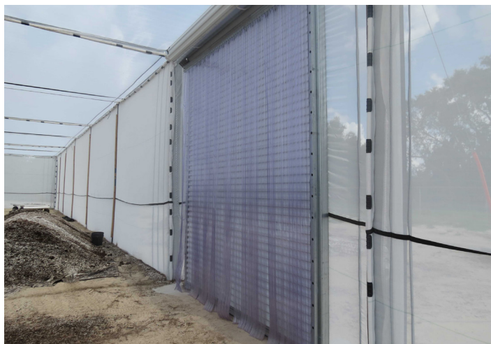
Figure 2. Steel roll-up door with a second plastic strip door, inside the CREC CUPS.
