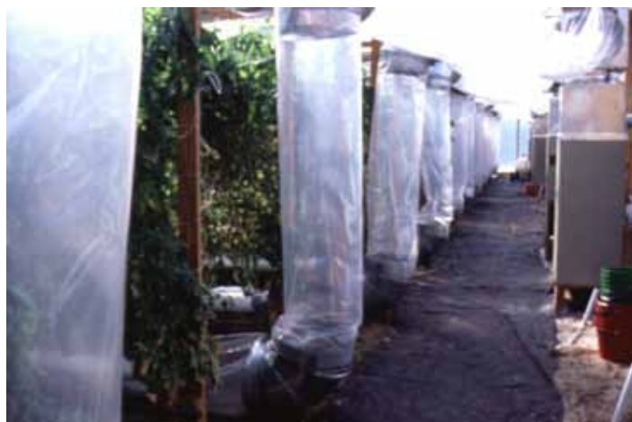
Figure 29. Distributing heated air on the floor helps warm the root zone and reduces condensation on the leaves and fruits.
