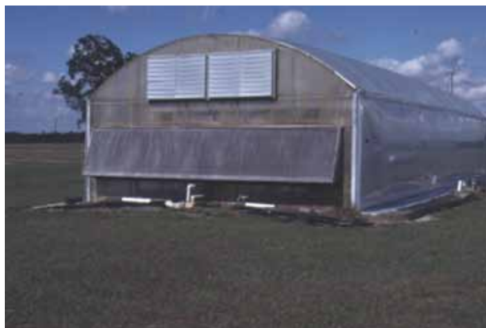
Figure 30. Motorized inlet shutters for winter ventilation.
