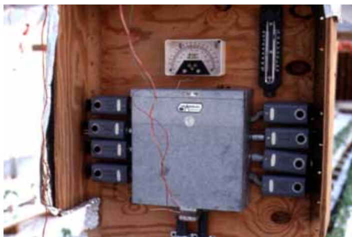
Figure 11. Panel board with thermostats that control greenhouse environmental system.
