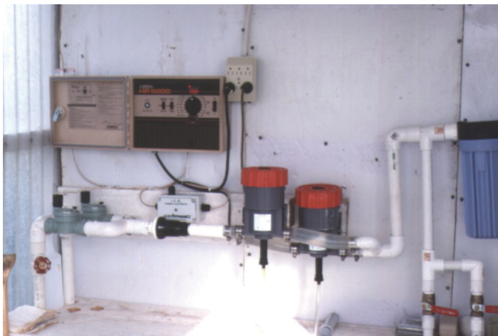
Figure 4. Irrigation controller, solenoid valves, pressure regulator, and proportioners for rockwool or perlite systems.
