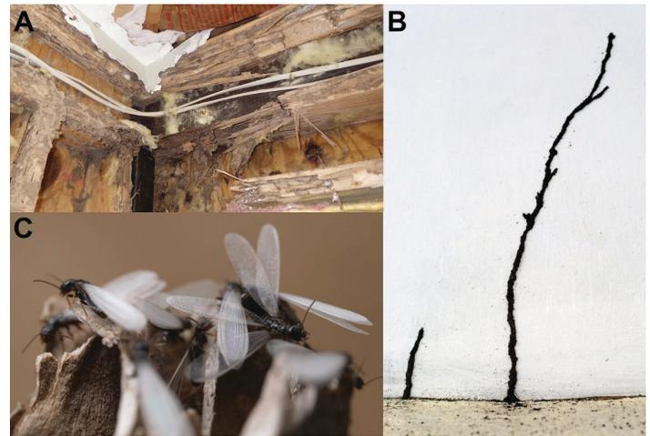
Figure 3. A) Extensive damage from *Reticulitermes flavipes* in a structure, discovered upon removing drywalls during remodeling. B) Mud tubes from *Reticulitermes flavipes*, coming from the ground. C) Dispersal flight event of *Reticulitermes flavipes*, with the emergence of winged individuals (alates).
