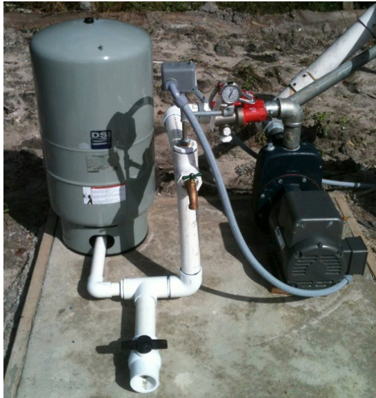
Figure 2. Pressure tank, 5-hp pump, 2" galvanized drop pipe, and red cycle stop valve.
