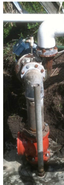
Figure 1. The 2" drop pipe (galvanized) installed below red check valve of original 6" well.
