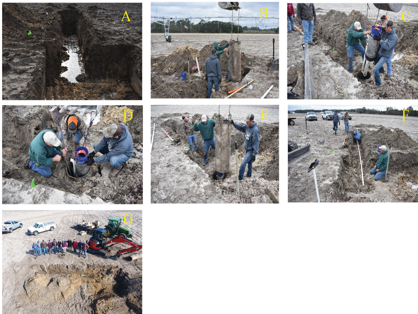
Figure 8. Installation of drainage lysimeter in UF/IFAS NFREC—Suwannee Valley, Live Oak, FL. A) Groundwater table visible. B) Inserting steel pipe to prevent soil from collapsing. C) Installing drainage lysimeter four feet below the soil surface. D) Drainage lysimeter within the steel pipe to keep the soil intact during lysimeter installation. E) Removal of the steel pipe after drainage lysimeter installation. F) Installing the PVC access pipes with the sensor cable and the sampling tube already inserted. G) An aerial view of the drainage lysimeter installation.
