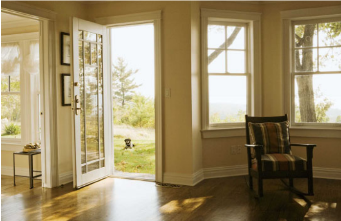
Figure 1. Check doors and windows to be sure they present no safety hazards.
