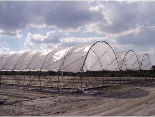
Figure 3. High tunnel with sides raised and ends open.
