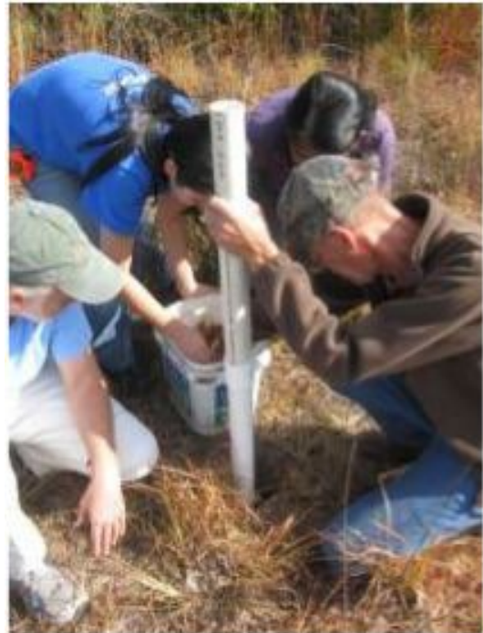
Figure 1. Citizen scientist volunteers assist in the installation of groundwater monitoring wells.
