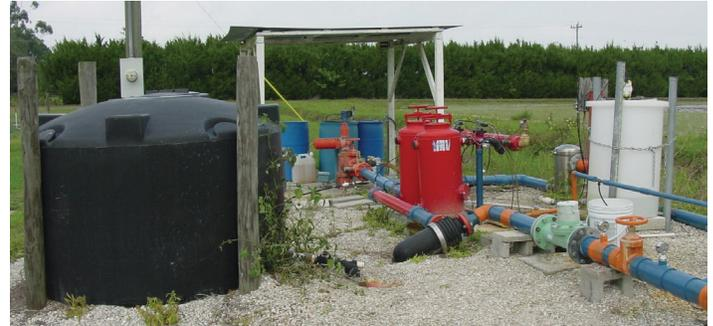
Figure 2. Fertigation equipment, including fertilizer tank (left), filters (center), and injector (right).
