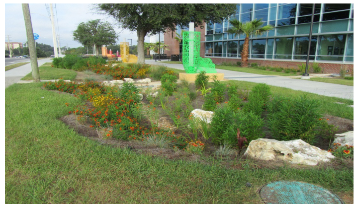
Figure 2. A bioretention area at SW Recreation Center, University of Florida Credits: Program for Resource Efficient Communities, University of Florida 2004
