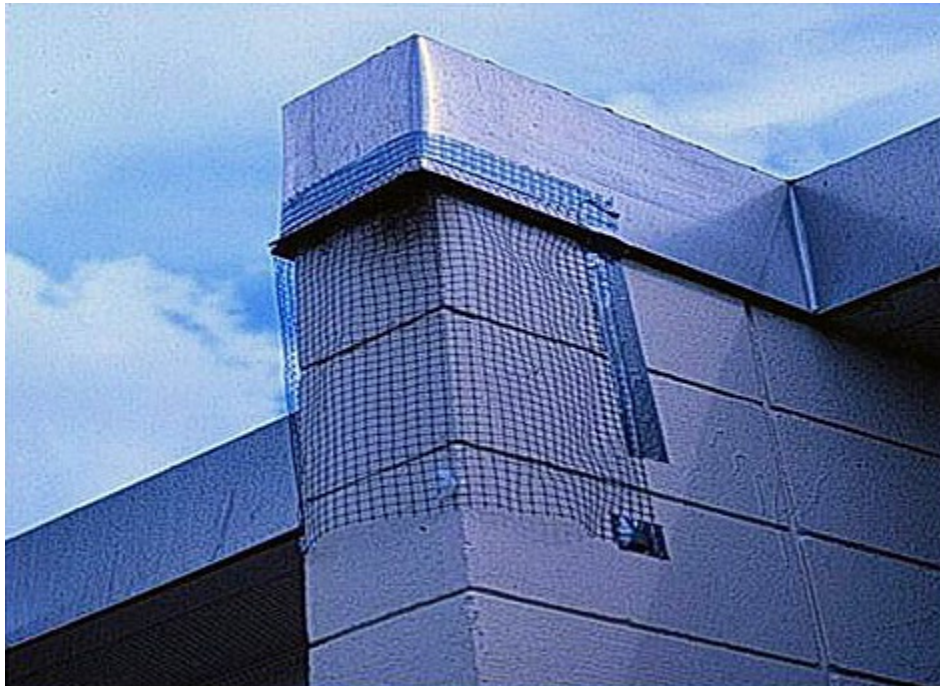
Figure 14. Devices, such as bat netting, can be placed where birds or bats reside to allow one-way movement out of the cavity, thus they can also be used for exclusion.
