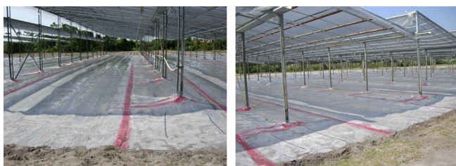
Figure 5. Overview of structure showing need to glue plastic for application to wide areas and to accommodate post rows.
