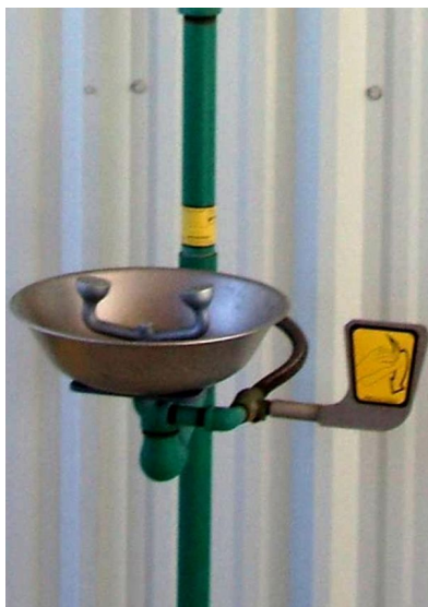
Figure 10. Plumbed eyewash station
