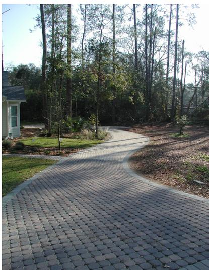
**Figure 9.** Pervious pavement installed for a driveway (Madera, Gainesville, FL). Credits: Mark Hostetler
