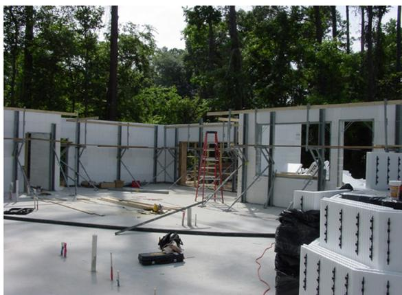
**Figure 7.** An example of Insulating Concrete Forms (ICF) used in residential construction. ICF is concrete poured into a type of foam mold with steel framing. This construction is sturdy and energy efficient. Credits: Hal Knowles
