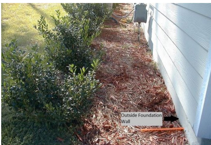
Figure 14. This home has maintained an excellent inspection space between the siding and mulch. Landscape plants are also positioned far enough away from the outside foundation wall to decrease moisture close to the home, and the placement accounts for future growth. Moisture is a conducive condition that can void some termite warranties. Credits: Faith Oi, UF/IFAS
