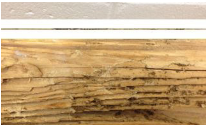
Figure 28. Subterranean termite feeding damage along the grain of the wood.
