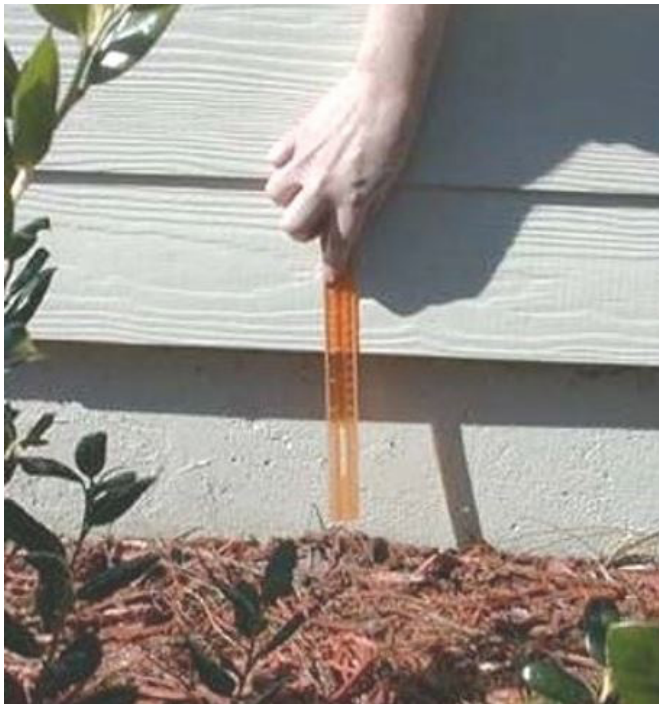
Figure 10. Building codes in many states require at least a 6-inch inspection space at the time of construction. It is important to maintain this inspection space and not hide it with mulch. When inspection spaces are obscured by mulch or other landscape plants, subterranean termites can access structures.
