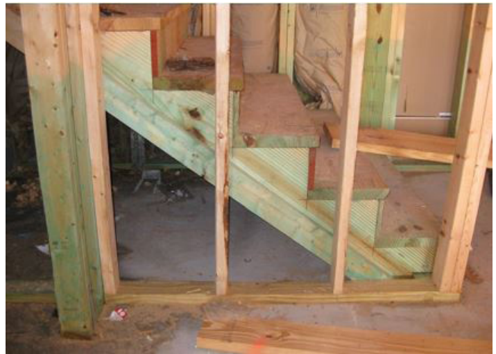
Figure 40. The dye marker shows that some wooden elements were treated, but the wall framing unit has likely been added since the treatment and is vulnerable to termites.
