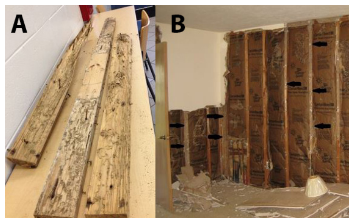
Figure 31. A) Subterranean termite damage in a room; B) Termites are blind, soft-bodied insects, so they follow guidelines, including wall studs. Arrows denote areas of prominent mud tubes.
