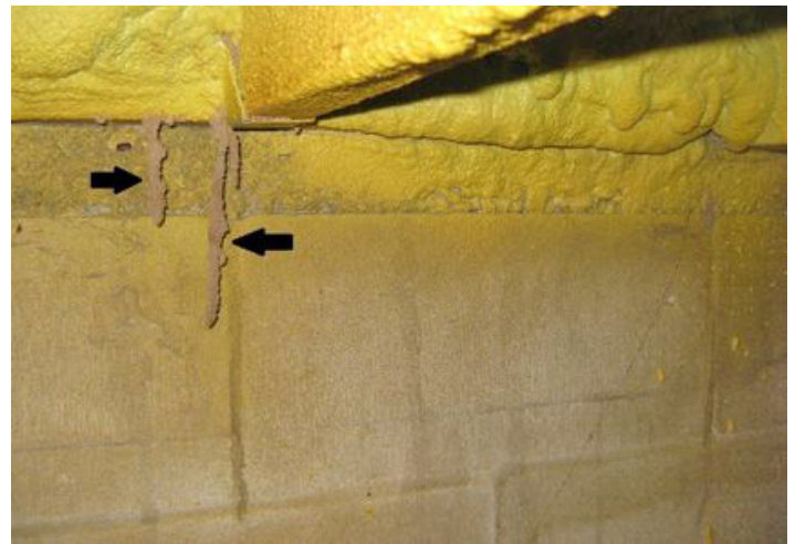
Figure 4. Arrows denote subterranean termite mud tubes emerging from behind spray foam insulation installed over floor joists in crawlspace.
