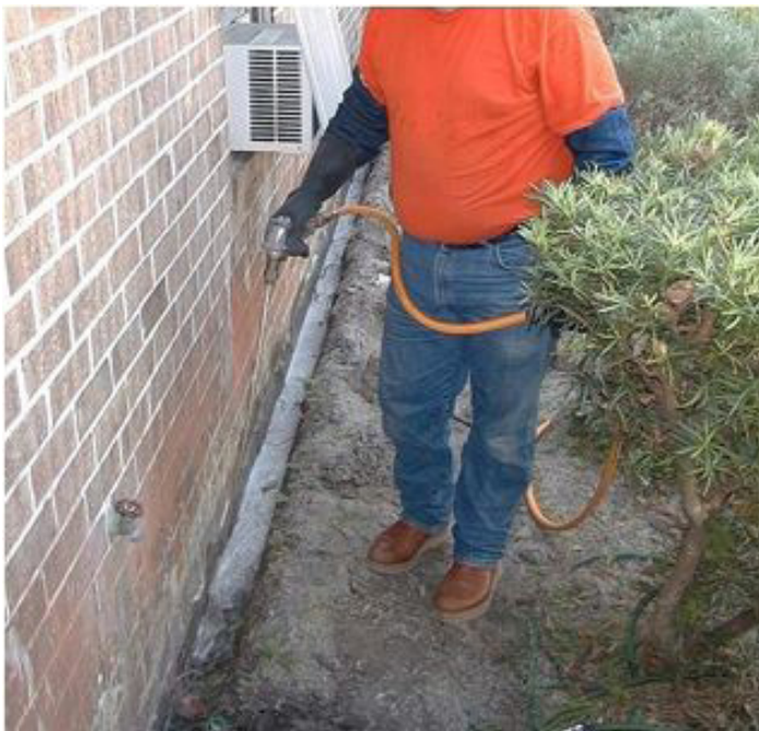
Figure 36. Applying the correct amount into the trench and drill holes requires that the pest management professional know how much termiticide is being sprayed at the end of the wand. They should have a rough idea of how many gallons per minute is being sprayed.
