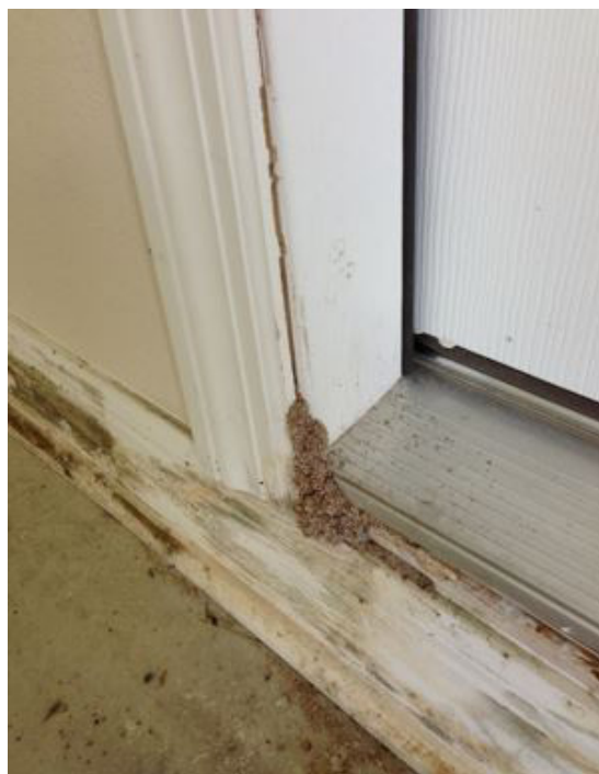
Figure 30. Subterranean termite mud tube at garage door baseboard and door frame, a common entry point.
