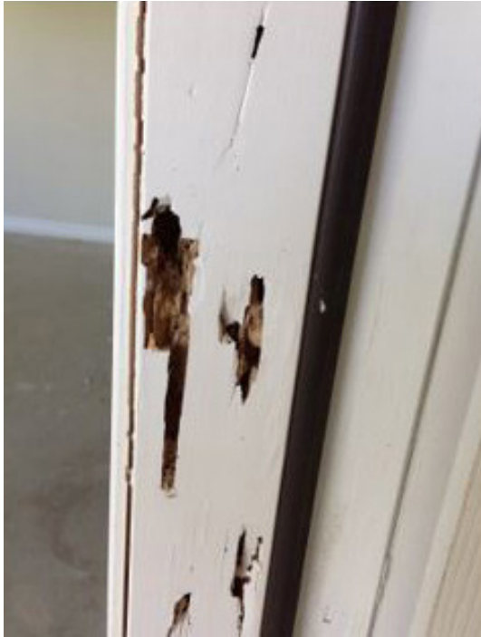
Figure 2. Termite damage on a door frame. Door frames are common access points. Doors often sit on expansion joints that allow subterranean termites to find their way in.
