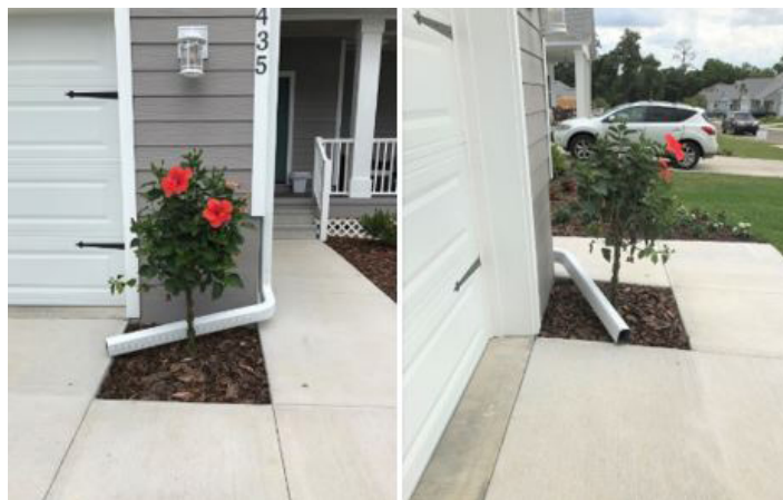
Figure 15. Improper plant placement and poor gutter placement. This newly planted hibiscus is one foot away from the home, but the branches are already almost touching the wall. Credits: Faith Oi, UF/IFAS
