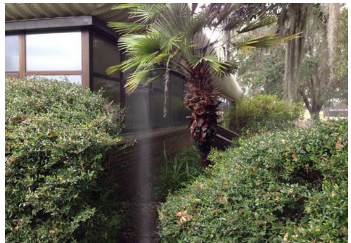
Figure 12. Irrigation head improperly directed, resulting in walls being watered. Wet walls create a conducive condition that will allow termites to thrive.
