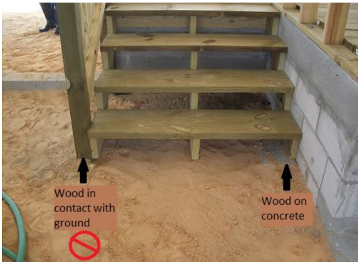
Figure 9. Example of wood-to-ground contact. Other examples in homes that may have wood-to-ground contact include piers, posts, attached fences, and decks. In this picture, the part of the wooden stair that is on the concrete pad may gain slightly more protection, but termites can still find the stairs via the gap against the wall.
