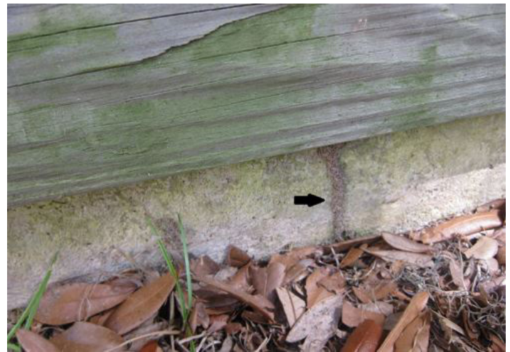
Figure 11. Termite tube that was detected on outside foundation wall that had an inspection space.
