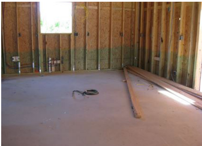
Figure 39. Borate-treated wall with a dye marker that shows where the treatment was applied.
