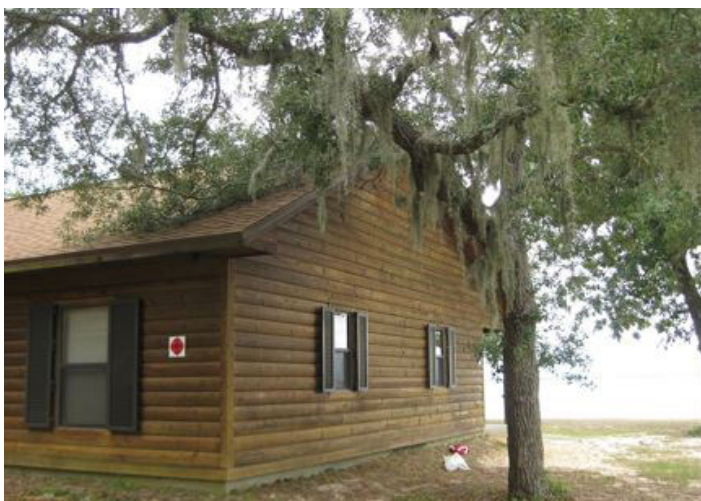
Figure 17. NO! The branches resting on the roof of this structure likely provided access for the Formosan subterranean termites that were found infesting the room below them.
