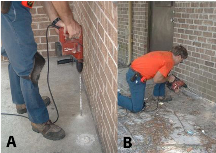
Figure 35. A) Down-drilling the slab so that termiticide can be injected under the slab and cut off subterranean termite access; B) Angle-drilling the slab. Another method to inject termiticide under the slab. Your pest management professional must understand building construction in order to know that the drill will emerge under the slab.
