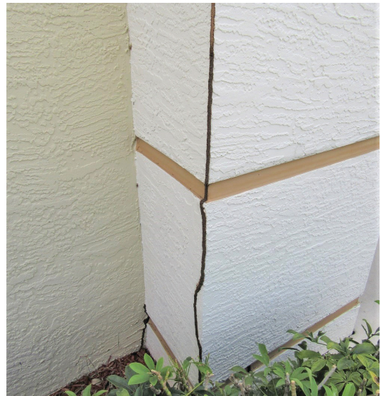
Figure 8. Nasutitermes corniger (Motschulsky) tunnel on the outer wall of a structure. Credits: Katherine Tenn, Florida Department of Agriculture and Consumer Services
