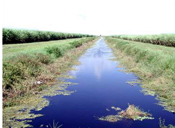
Figure 10. Stabilization of canal banks with vegetation.
