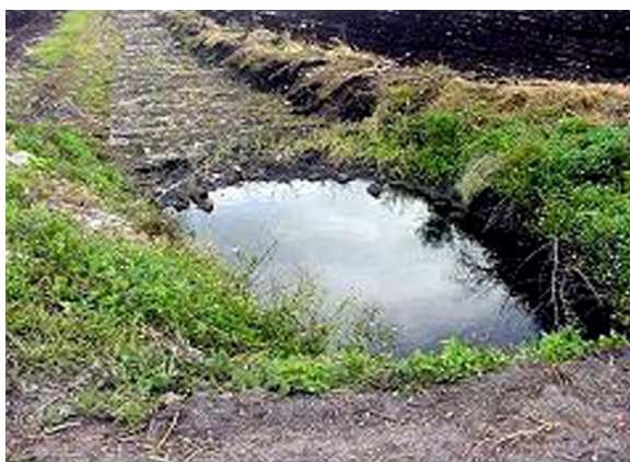
Figure 5. Typical field ditch sediment sump.
