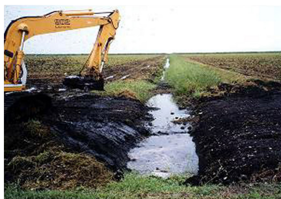
Figure 6. Removal of soil and sediment buildup in field ditches.
