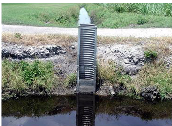
Figure 7. Riser boards slow drainage near pumps.
