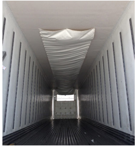
Figure 9. Interior view of refrigerated trailer showing flat sidewalls, duct extension, air delivery chute, pressurized return air air bulkhead, a duct extension, and an air delivery chute attached to the ceiling of a reefer trailer. (Source: PEB Commodities, Inc.)
