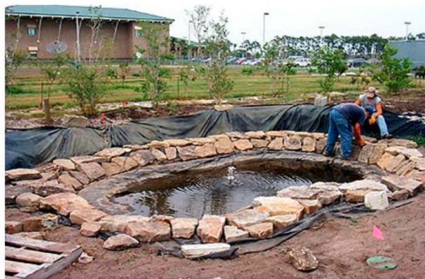
Figure 3. Installation of pond structure in IRREC ornamental teaching gardens.
