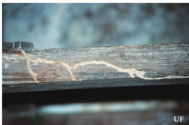
Figure 13. Heterotermes subterranean termite foraging tube on a sheltered bench, Cat Island, Bahamas. Credits: Rudolf H. Scheffrahn, University of Florida
