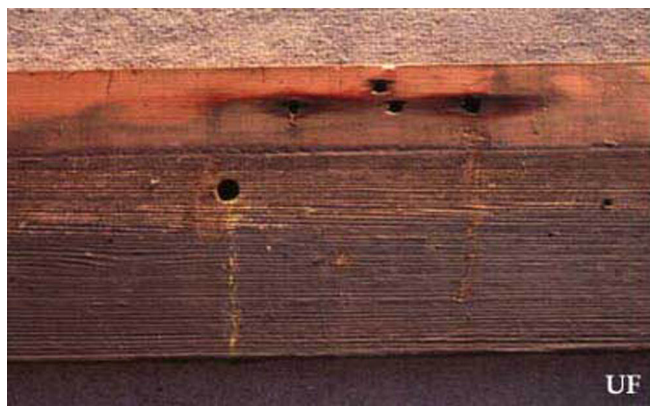
Figure 6. Entry hole drilled into structural wood by a large carpenter bee, Xylocopa sp. Credits: University of Florida
