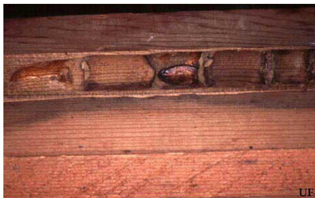
Figure 7. Internal damage to structural wood by a large carpenter bee, Xylocopa sp., showing individual larval cells. Credits: University of Florida
