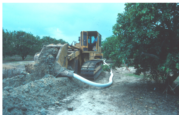
Figure 8. Horizontal well installation.
