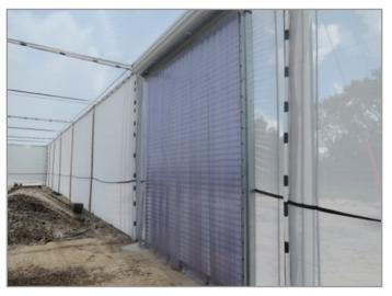
Steel roll-up door with a second plastic strip door, inside the CREC CUPS
