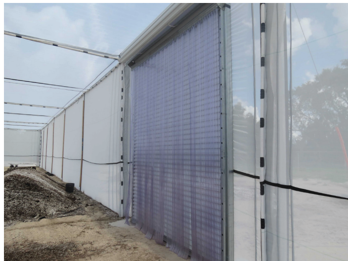
Figure 1. Steel roll-up door with a second plastic strip door, inside the UF/IFAS CREC CUPS.
