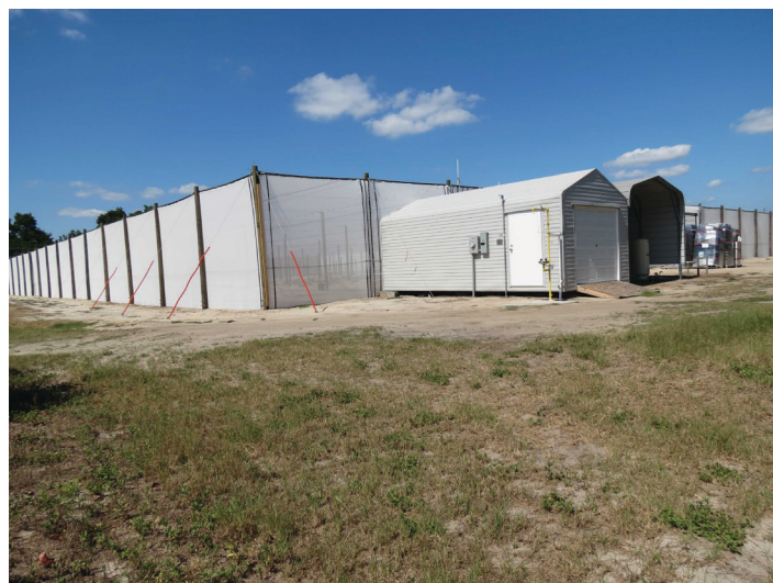
Figure 3. The UF/IFAS CREC CUPS facility near Lake Alfred, FL.
