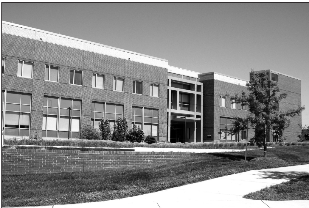
Figure 1. The BTEC facility on NC State's Centennial Campus.
