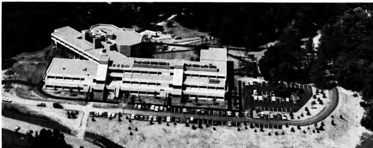
Clarkson's multimillion dollar Science Center was dedicated in 1970 and is one of the finest facilities of its kind in New York.
