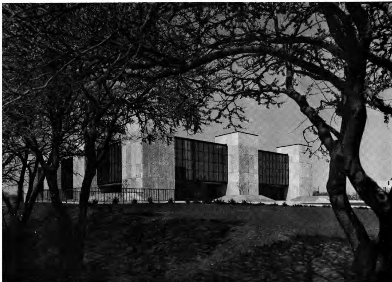
DURLAND HALL—New Home of Chemical Engineering
