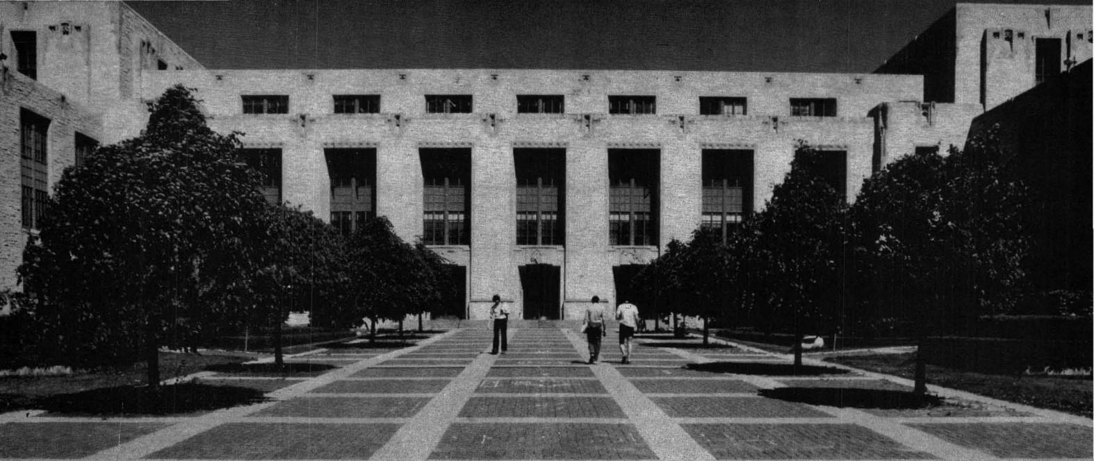
The Technological Institute, home of the Department of Chemical Engineering.
