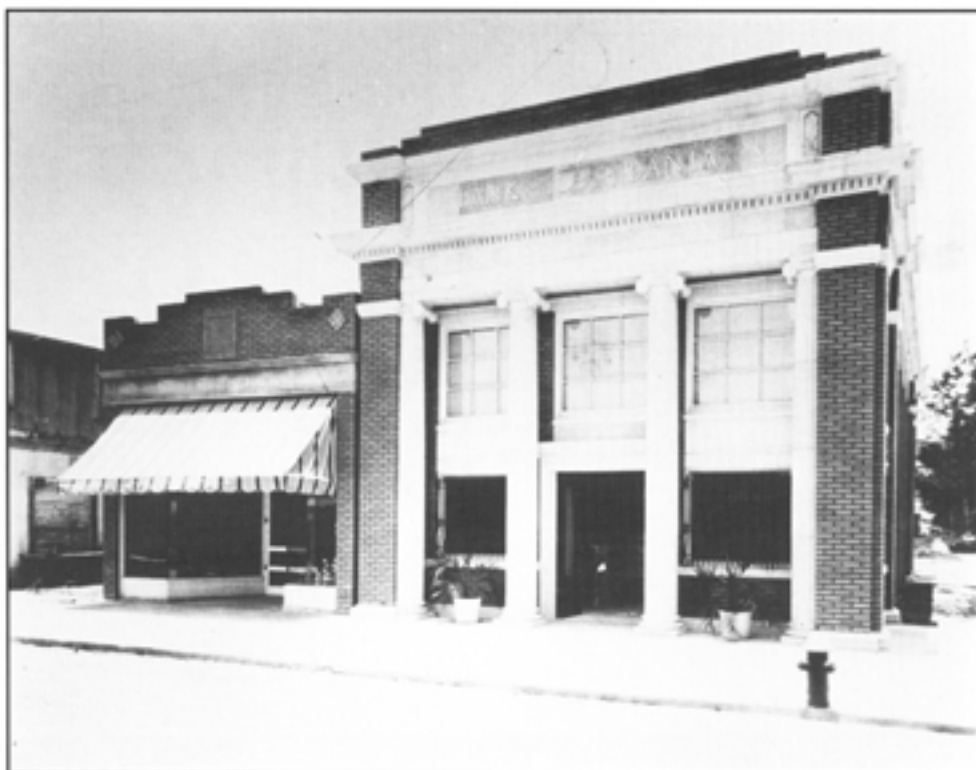
Dania Bank Building, built 1924 Federal Highway and Dania Beach Boulevard, Dania Beach The city's only bank until 1956, this fine Neo-Classical style building could probably be listed in the National Register.
