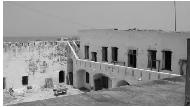
Figure 2. Engineer: John Apperley (English), European and Fante Builders, interior Fort William, 1753-1759, local and imported bricks, local stone, imported lime, Anomabo, Ghana. Author's photograph.
