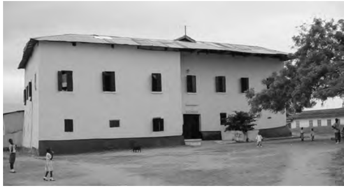
Figure 1. Designer: Heindrick Caerlof (Polish), European and Fante Builders, Dutch Lodge/Omanhene's Palace, c. early 1640s, imported bricks, local stone, imported lime, Anomabo, Ghana. Author's photograph.
