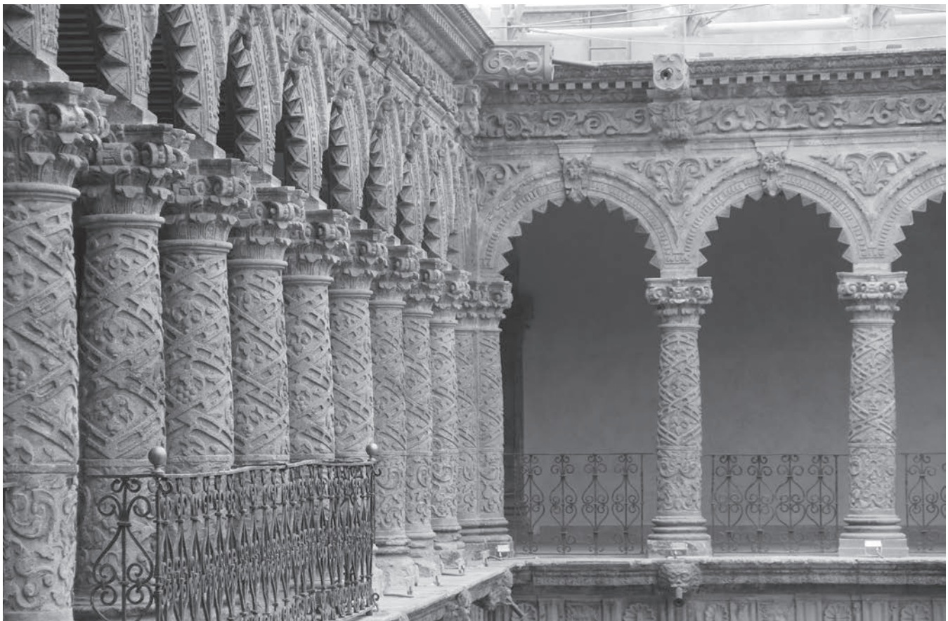
Figure 3. Detail of diamond rustication within the polylobed arches of Claustro de la Merced, c. 1676-1703, Mexico City, Mexico. Photo credit: Martha Lara Vázquez.
