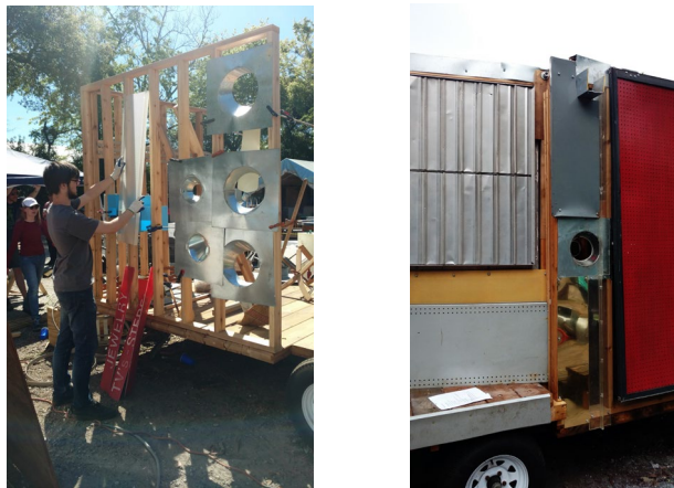
Figures 1 and 2. Found building materials led to innovative cladding solutions. © Ana McIntosh
